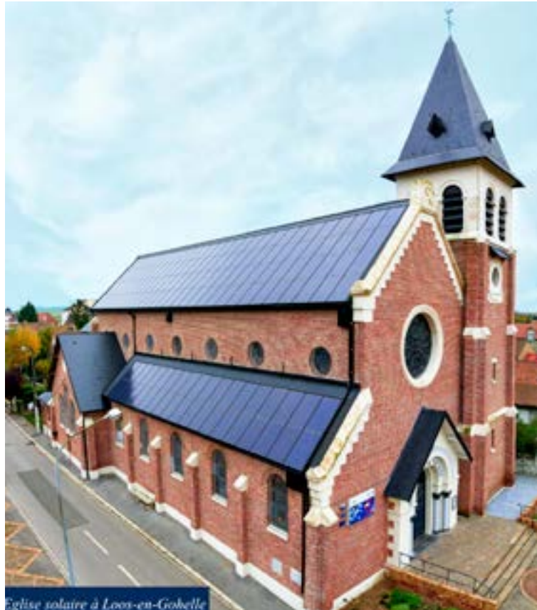
The town's church, equipped with solar panels
